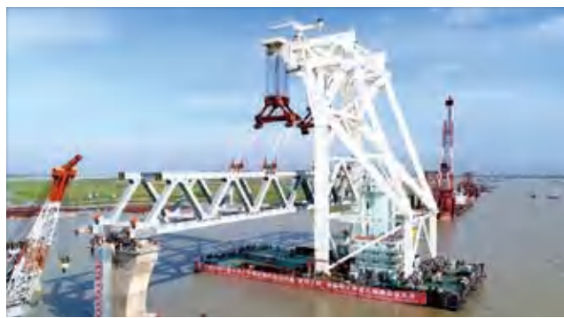
孟加拉国“梦想之桥”——帕德玛大桥架设主桥钢梁 Main bridge steel beams were erected on the “Bridge of Dreams”, the Padma Bridge, in Bangladesh
