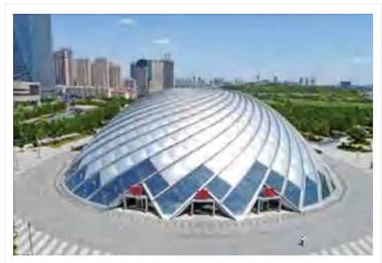
滨海站站房外正立面 The facade of the station building of Binhai Station
